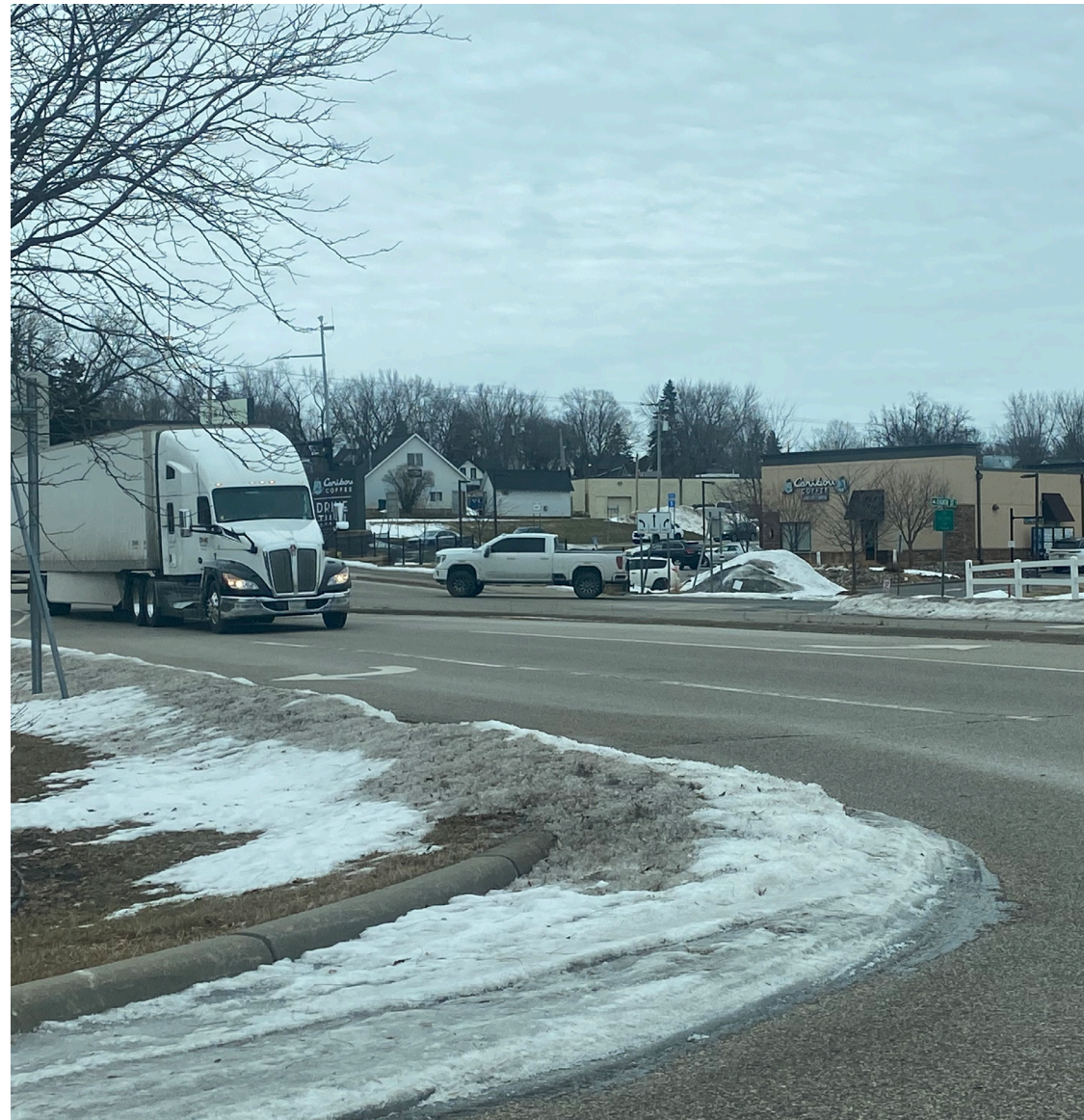
Walgreens access facing northeast
