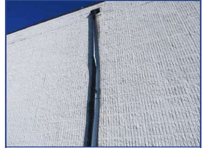
Damaged downspout
