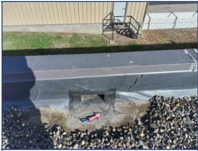
Deteriorated Flashing
