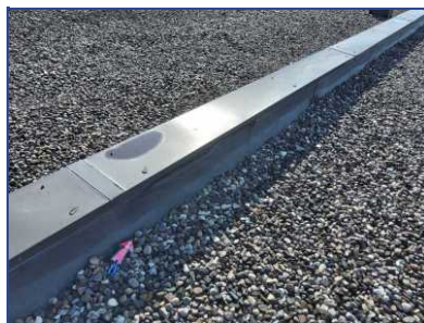
Membrane Shrinkage
