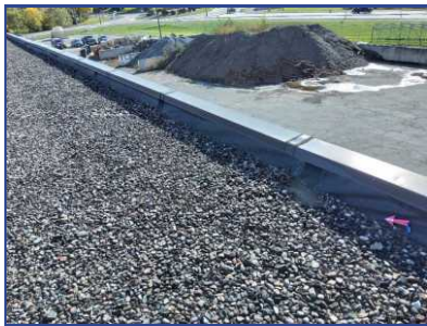
Membrane Shrinkage
