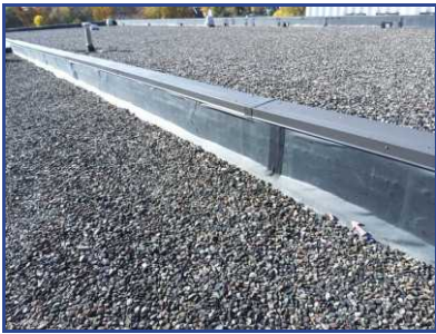
Membrane Shrinkage
