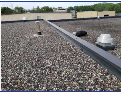
Membrane Shrinkage
