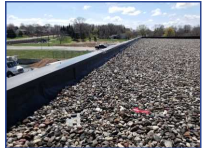
Section A - Def 3 - Before Photo
