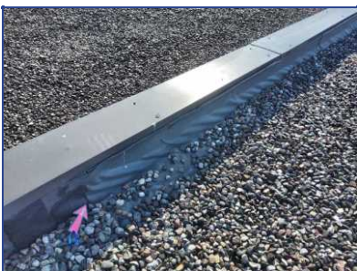
Membrane Shrinkage
