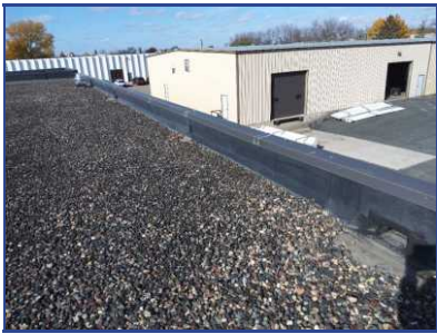
Membrane Shrinkage
