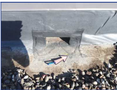
Deteriorated Flashing
