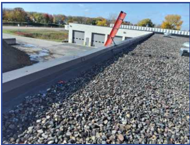
Membrane Shrinkage
