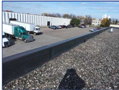
Membrane Shrinkage
