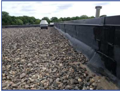
Membrane Shrinkage
