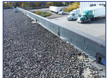
Membrane Shrinkage
