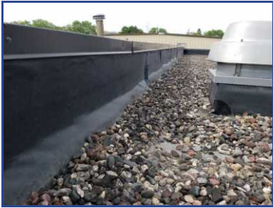
Membrane Shrinkage
