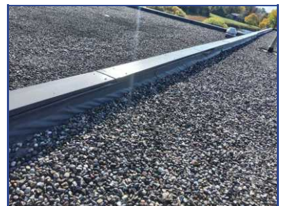
Membrane Shrinkage
