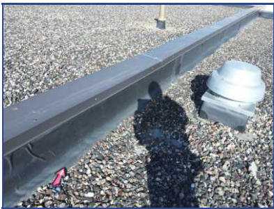
Membrane Shrinkage
