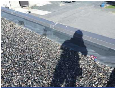
Membrane Shrinkage
