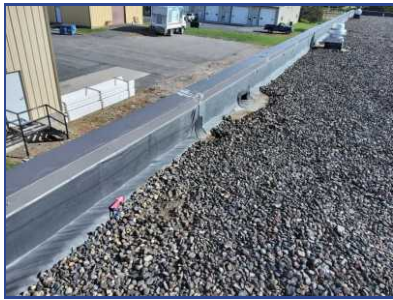
Membrane Shrinkage
