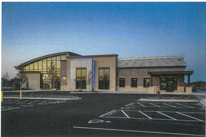
SOUTH ELEVATION VIEW OF TCO FROM PARKING LOT - LOCATED NORTH OF PROPOSED SITE
