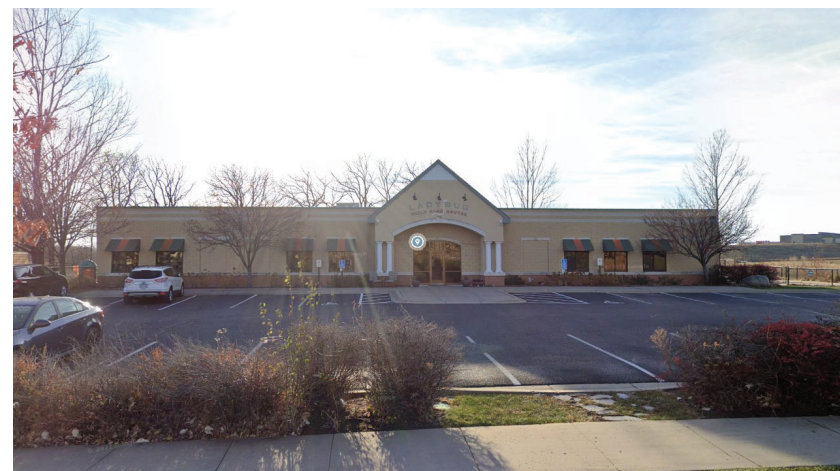
EASTERN NEIGHBORING BUILDING - LADYBUG CHILD CARE CENTER
