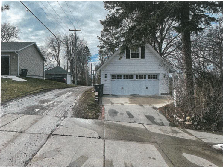
Neighbor detached garage at 40 Pine St
