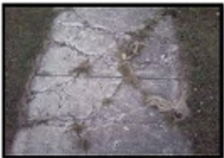
Cracking
