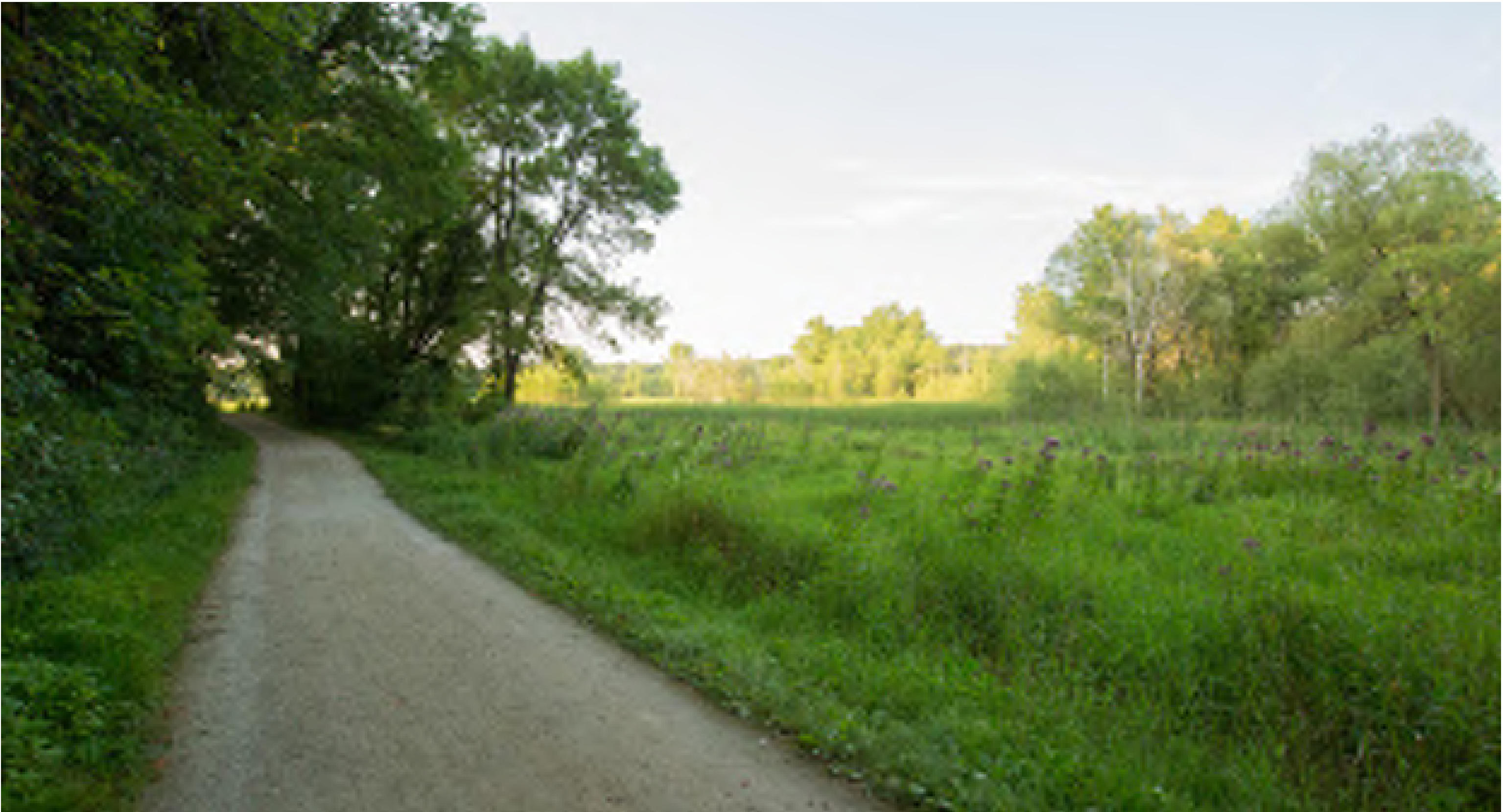
SECONDARY TRAIL (CRUSHED LIMESTONE CONSTRUCTION (5’ WIDE))
