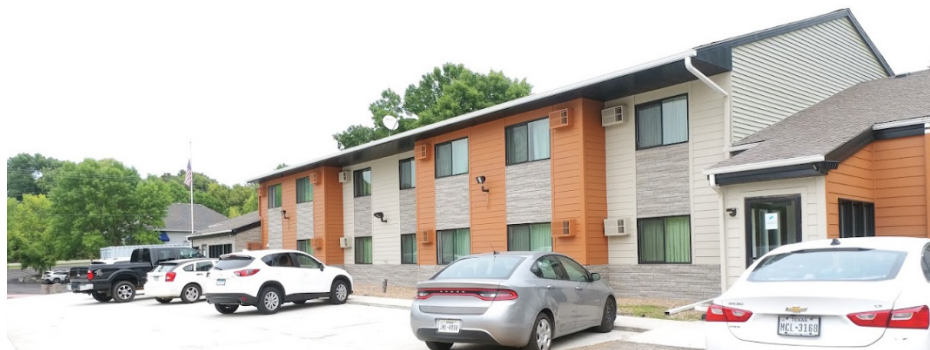
WACONIA INN & SUITES 301 E FRONTAGE RD
