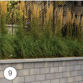
Retaining Wall Planter
