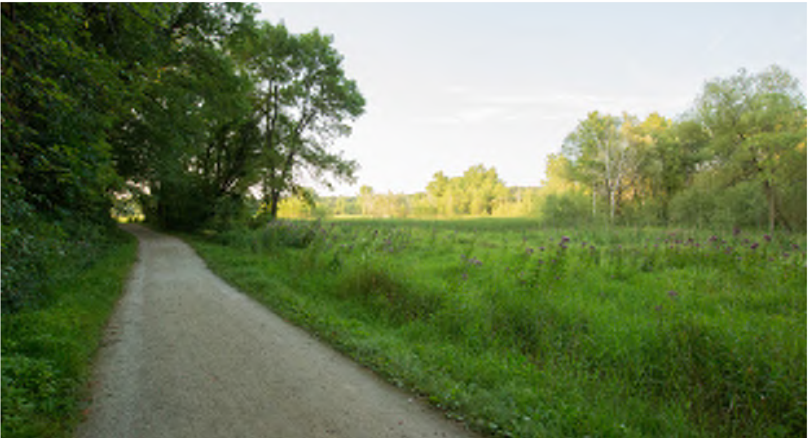
SECONDARY TRAIL (CRUSHED LIMESTONE CONSTRUCTION (5’ WIDE))
