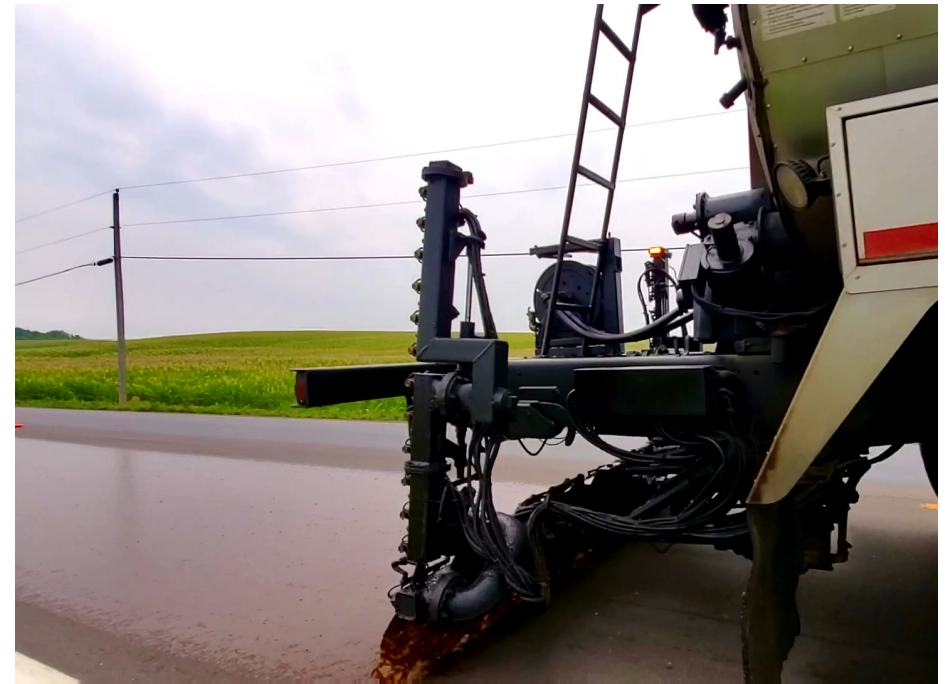
Application of SOR on an asphalt pavement
