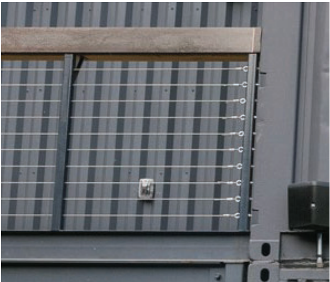
STEEL PROPOSE RAILING W/ WOOD POST CAP
